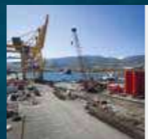
QUAY UPGRADE deepening, widening
